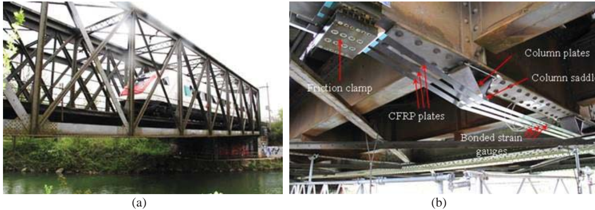
Figure 6. (a) Münchenstein railway metallic Bridge (120-year-old) subjected to a passenger train. The bridge consists of 10 panels with the total length of 45.2 m, width of 5 m and height of 6.15 m and built on a 45-deg skew. (b) The cross-girders were retrofitted with pre-stressed un-bonded CFRP strips (Ghafoori et al. 2015b).
