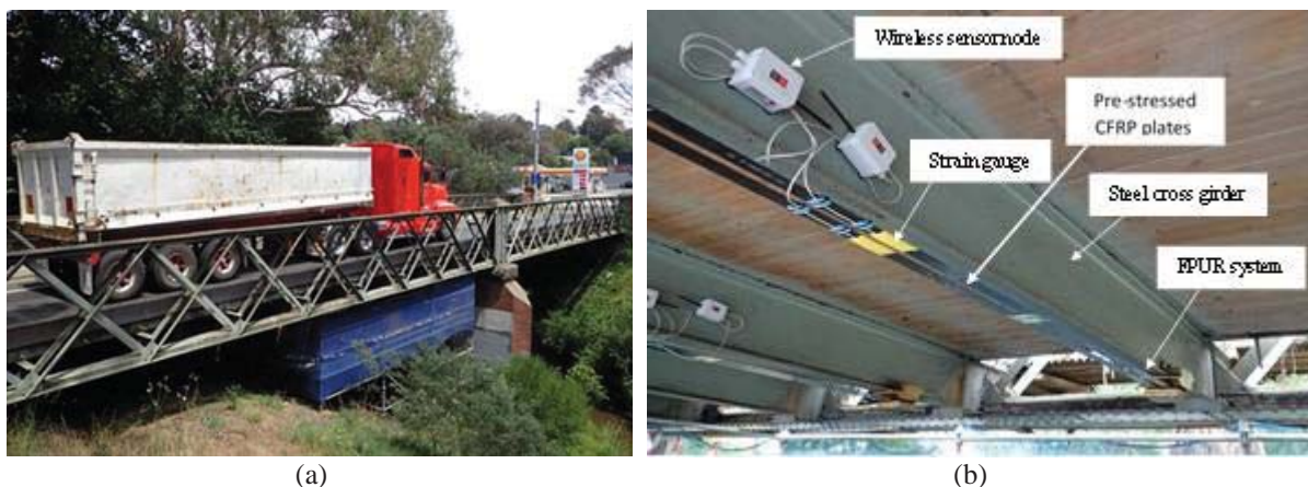
Figure 7. (a) Diamond-Creek Bridge, Melbourne, Australia, (b) application of the FPUR system for CFRP strengthening of the bridge cross-girders (Ghafoori et al. 2018).
