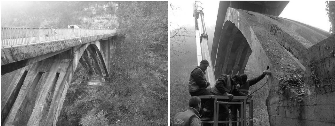
Figure 3. Roverè bridge: (a) view of the bridge; (b) test on the arches of the bridge.
