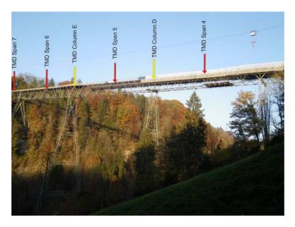
Figure 11, Positions of vertical (red) and horizontal (yellow) TMD's.
