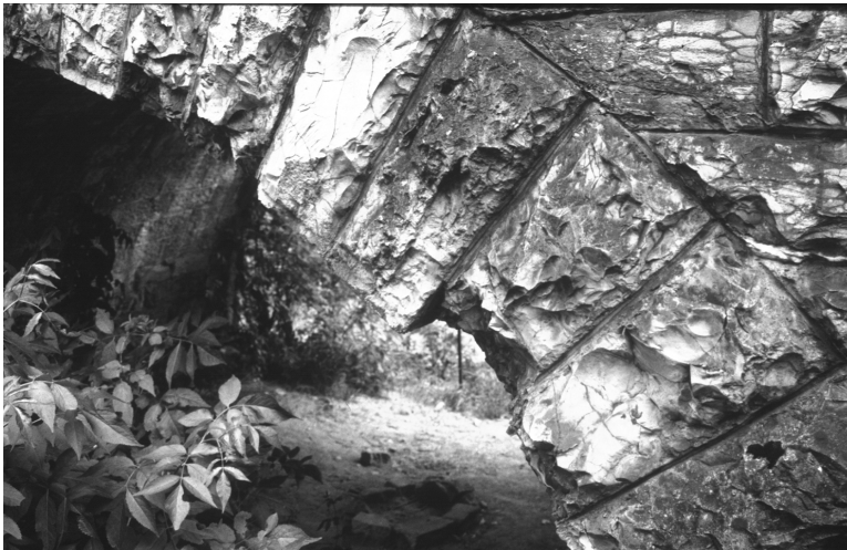
Figure 2: Crumbling decay on Jurassic limestone
