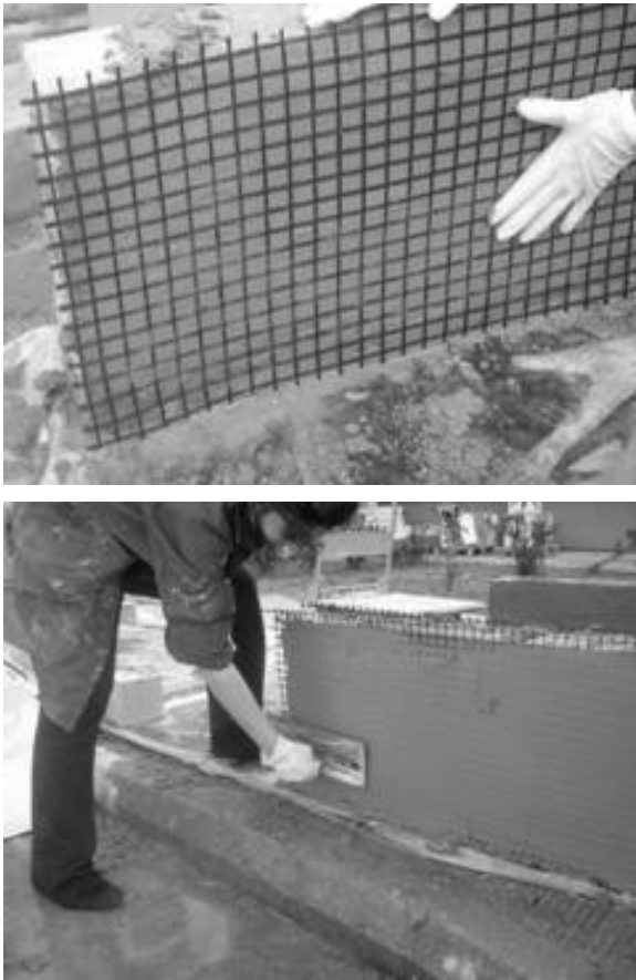
Figure 8. Application of RM Basalt system at the Structural Materials Laboratory in University of Patras (Operha Project).
