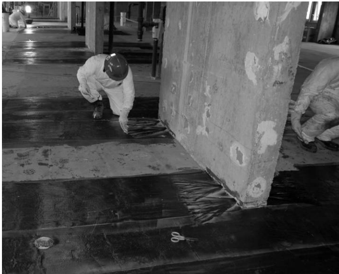
Figure 7. Anchorage through walls (Fyfe Company).
