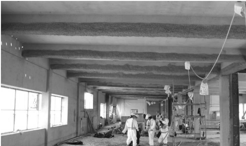
Figure 2. Application of AFP System on FRP strengthened beams (Fyfe Company).
