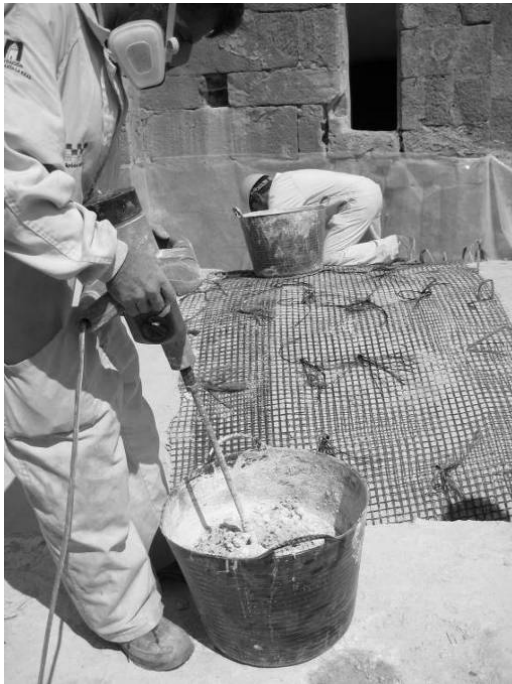
Figure 10: Strengthening a vault of a Romanesque church in Spain (Operha Project).
