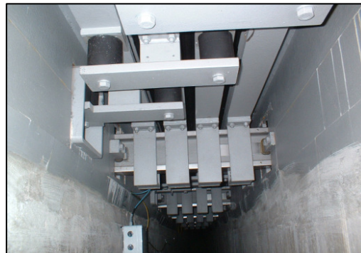
Figures 2 and 3. Load monitoring at bearing and movement monitoring at expansion joint.
