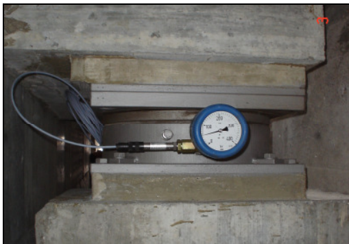
Figures 2 and 3. Load monitoring at bearing and movement monitoring at expansion joint.
