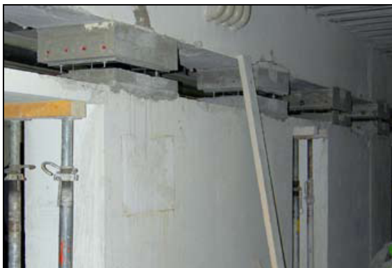
Figure 7. Sliding bearings inserted in internal basement wall
