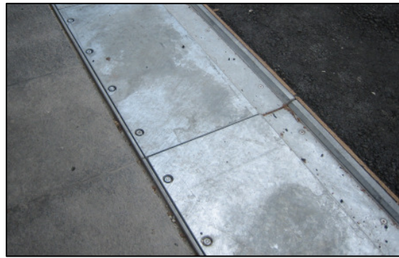
Figure 10. Installed expansion joint at vehicle exit
