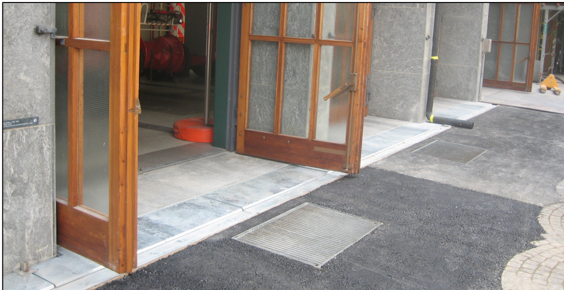
Figure 11. Vehicle exit point after completion of works, showing new stainless steel expansion joint
