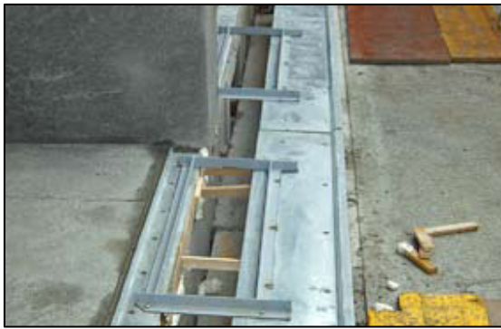
Figure 9. Installation of expansion joint
