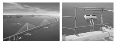
Figure 2. Incheon Grand Bridge (South Korea) with independent power supply for the monitoring system
