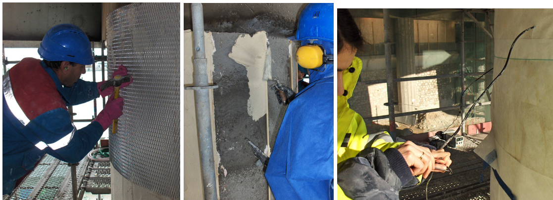
Fig. 4: anode installation, pulp installation, electrical connexions for the temporary chloride extraction system
