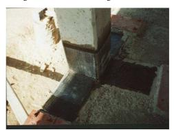
Column-beam connection by using FRP bands
