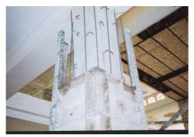
Installation of concrete jacket around column
