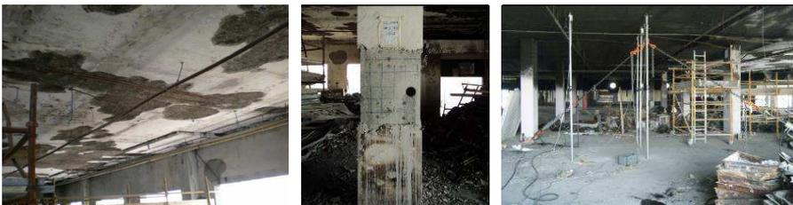
Figure 6. (a) Fire damages on the slab; (b) Concrete sampling at columns; (c) Static load test.
