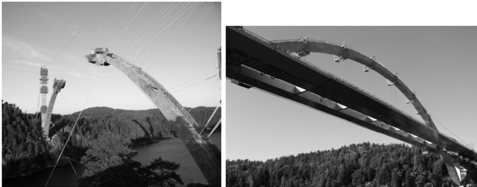
Figure 2. The New Svinesund Bridge joining Sweden and Norway. The main span is a single arch with a bridge deck on either side of the arch. Photographs of the bridge under construction.
