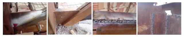
Figure 6. Some typical welding in the dormitory
