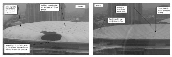
Figure 2: BC roof break (left) and deflation (right) [1]
