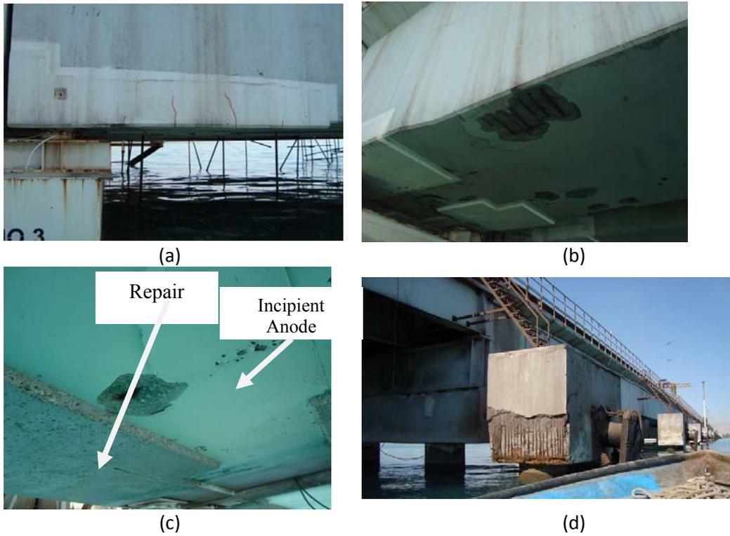
Figure 2- a) Crack occurrence in supporting points b) reinforcement corrosion under Channel bridge c) formation of incipient anode d) corrosion in fenders
