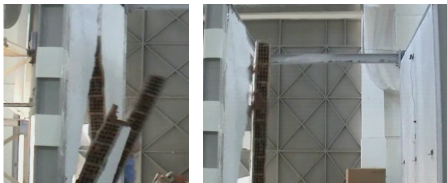
Figure 7. Collapse of the middle wall part (left), total collapse of the unreinforced wall and failure free reinforced wall (right)
