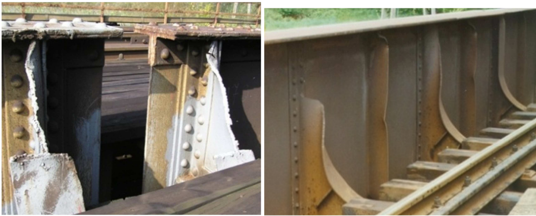
Figure 2. Typical defects of transverse intermediate stiffeners caused by the impact of vehicles crossing the bridge (Bień J., 2010)
