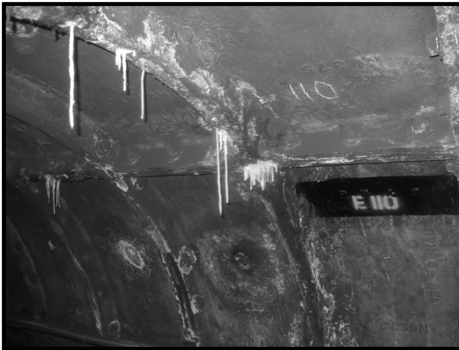
Figure 3. Staining, stalactite growth and rusting are seen in the joints.
