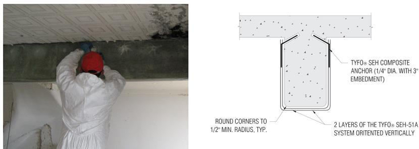
Figure 7. Application of anchors for shear strengthening of beam (courtesy of Fyfe Europe)
