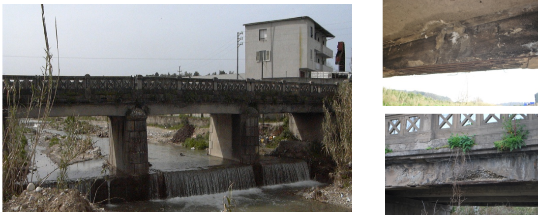
Figure 1. State of the bridge before retrofitting, general view and close-up views of the bridge deck.
