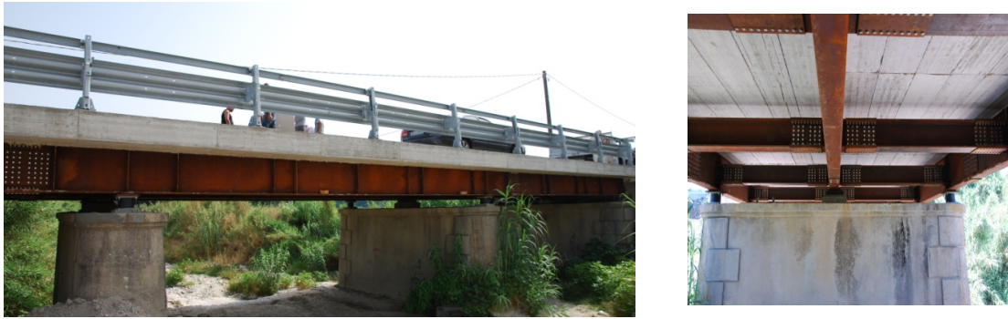
Figure 2. General views of the bridge after retrofitting (composite steel deck and HDR isolators and sliders).
