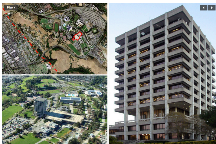
Figure 1. Location of the Hayward Fault and the Warren Hall
