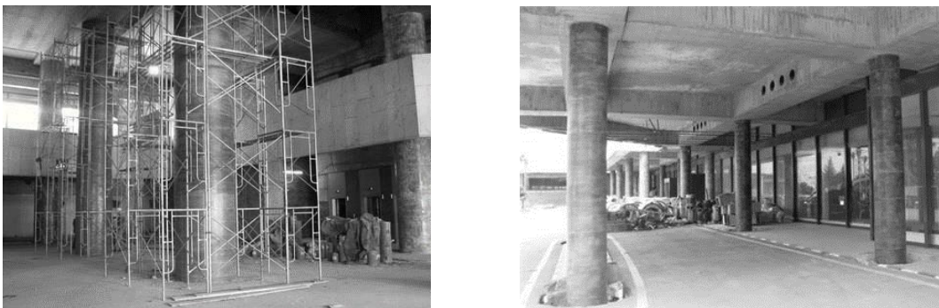
Figure 6: Hotel Parsian Azadi, Confining Columns using CFRP sheets
