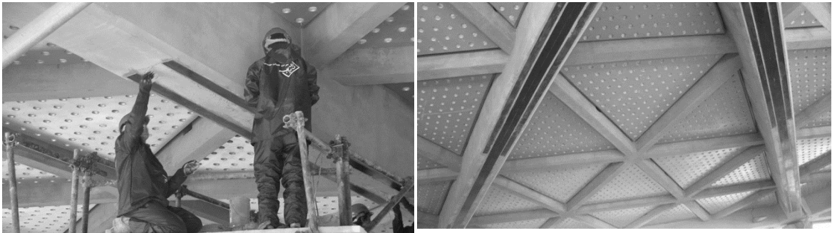
Figure 9: Qomrud Bridge, Concrete beams are strengthened using CFRP laminates
