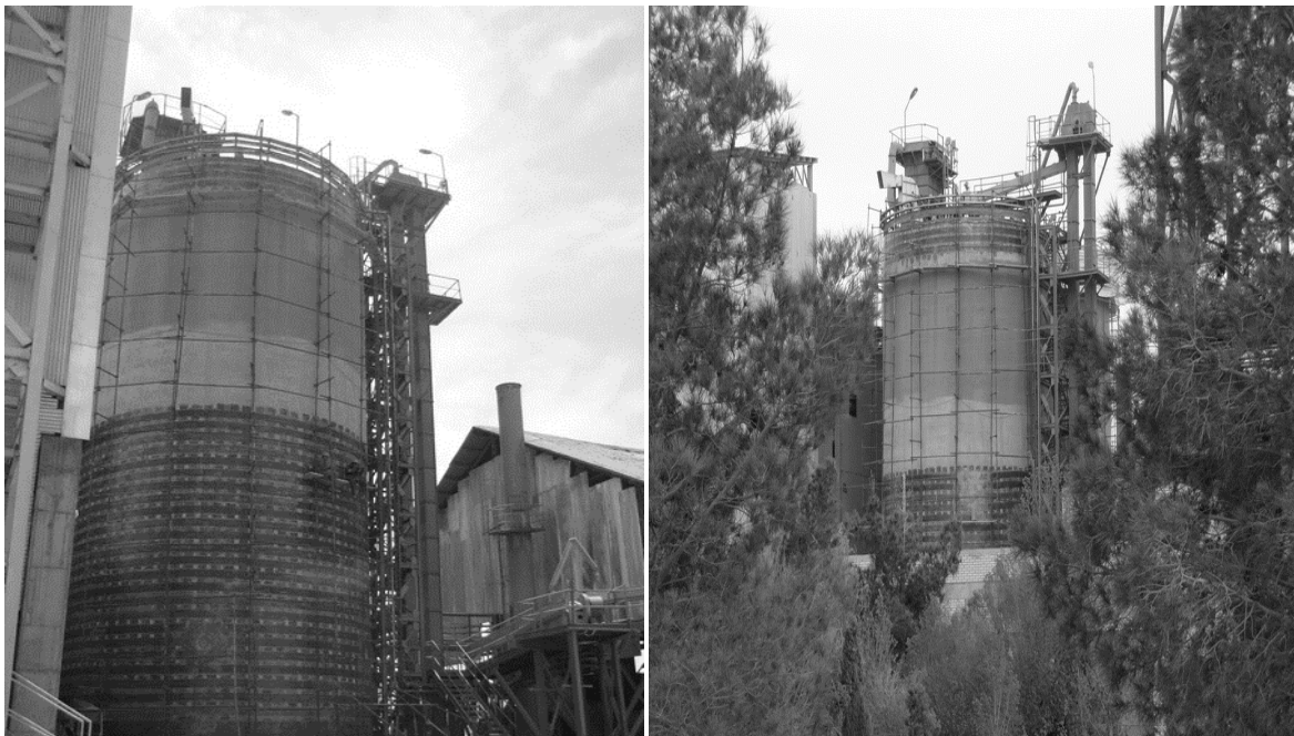
Figure 10: RC silos are strengthened using CFRP sheets in two perpendicular directions
