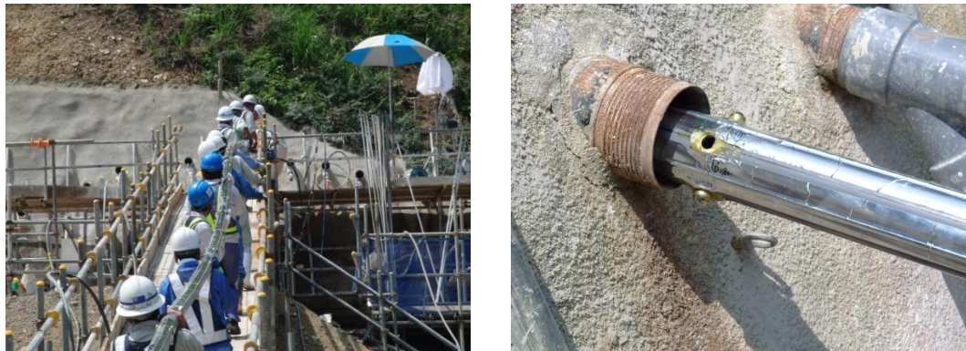
Figure 7. Smart rod installation process (left) and ELSP (right)
