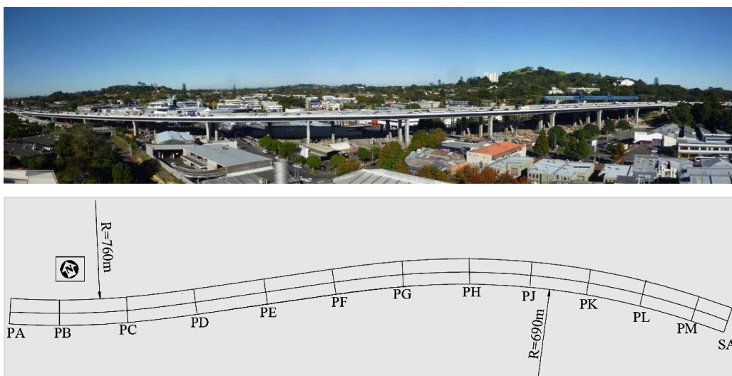
Figure 2. The view and plan of the Newmarket Viaduct in Auckland ( https://www.nzta.govt.nz/ ).
