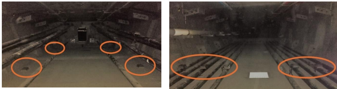
Figure 3. Bridge instrumentation using the wireless sensory system.
