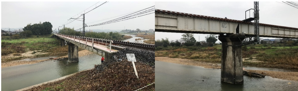
Figure 1. Photo of target bridge pier.
