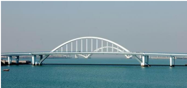
Figure. 1 Panorama of Tianyuan Bridge
