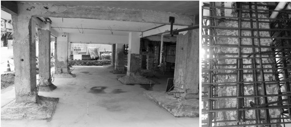
Figure 5. Process on foundation and columns.
