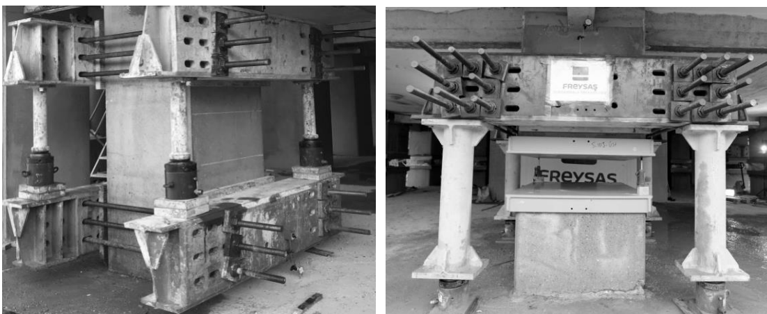
Figure 6. Clamp system.
