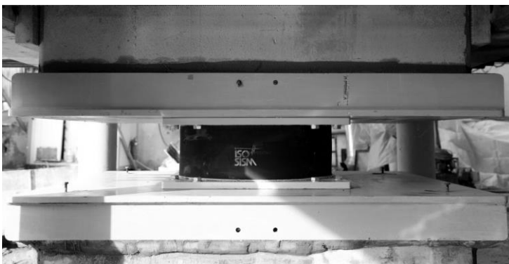
Figure 8. Installed isolator.
