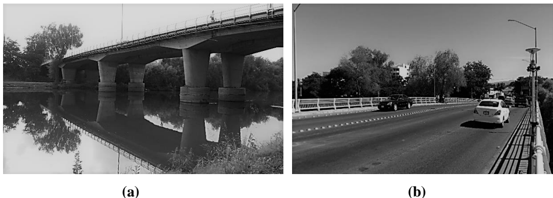
Figure 1. The Juarez Bridge: (a) Dimension and currently condition; (b) Location and fixing conditions of the GPS receivers.
