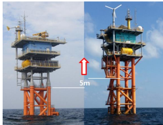
Figure 2. Gageocho ORS before and after recovery (Shim et al. 2015)
