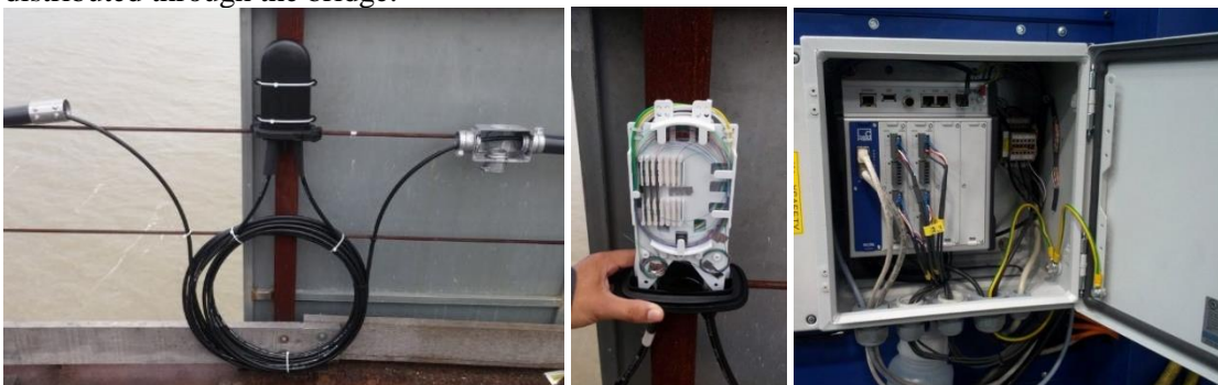
Figure 6. Multi-fiber cable splice protection box (left and center) and PMX device (right).
