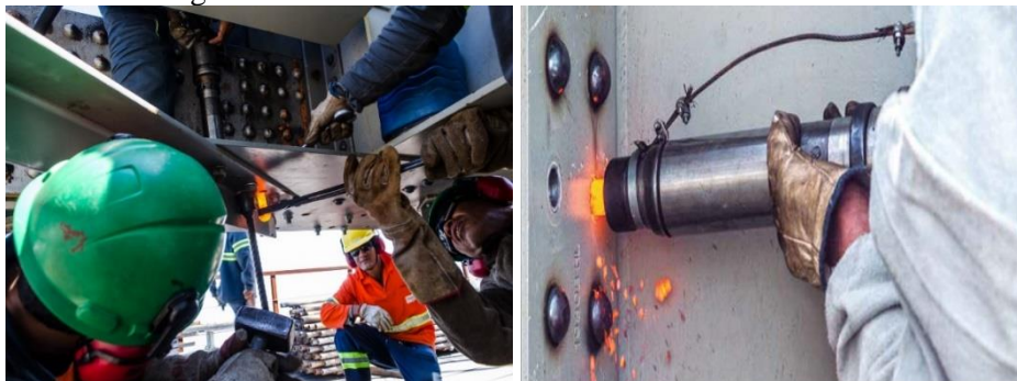
Figure 2. Attachment of rivets.
