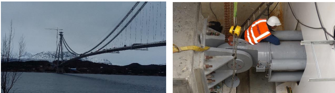
Figure 9. The Hålogaland Bridge (left), and installation of one Reston-STU shock transmission unit at a pylon to control deck movements – designed for axial force of 10,400 kN and with a stroke of +/-450 mm.
