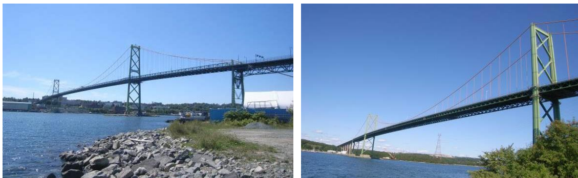
Figure 6. Angus L. Macdonald Bridge and A. Murray Mackay Bridge, Halifax, Canada.
