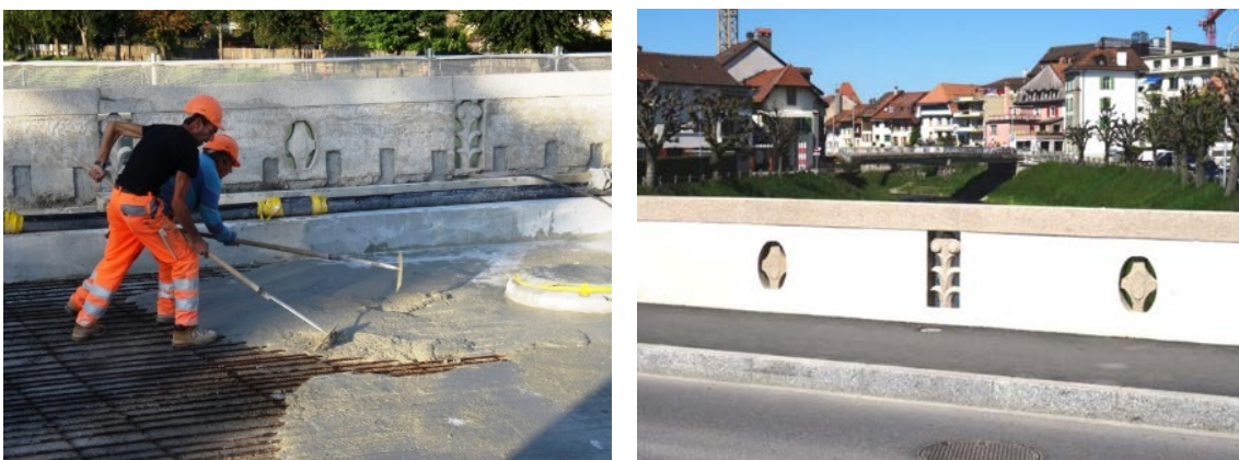
Figure 13. Casting of the UHPFRC on the deck slab; the UHPFRC layer incorporates steel rebars. Restored decorative elements of the parapets.
