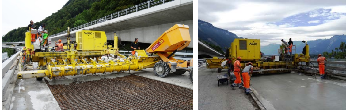
Figure 15. Casting of the UHPFRC using a machine.
