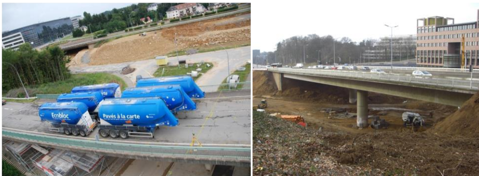
Figure 6 “Deutsche Bank bridge” (left) [11] and the “Champangshiehl bridge” (right) [12]
