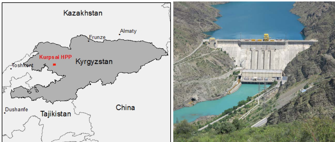
Figure 1. The Kurpsai Hydropower Plant (HPP) and its surroundings (right; Photo © M. Pilz) as well as the location in the Kyrgyz Republic (left).
