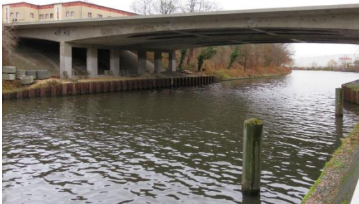
Figure 4. Side view of the Sieversbrücke.
