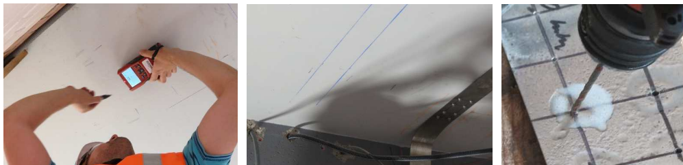
Figure 2. Preparation of laminates and concrete surface
