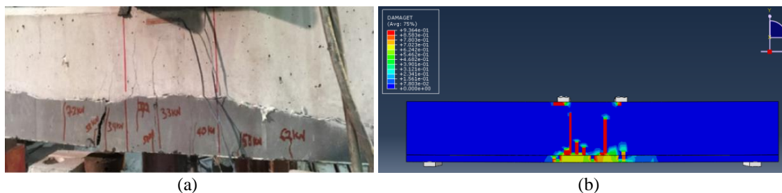
Figure 9. Crack pattern for the strengthened RC beam (a) experiment (b) 3D-Cohesive FEM
