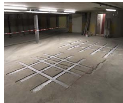
Figure 6. Heating process with infrared heating units (left), strengthened RC slab before grouting (right)
