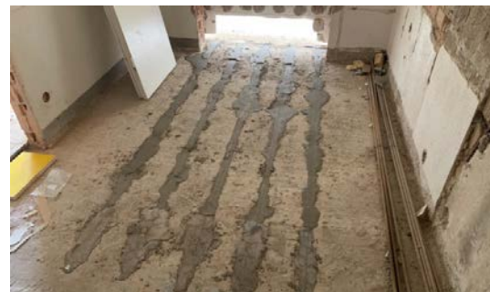
Figure 11. Activation of end-anchored re-bars with infrared heating units (left), RC slab, strengthened with near-surface mounted re-bars (right)
