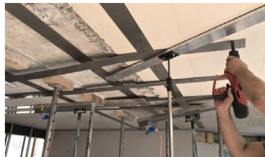
Figure 8. Hospital, Thun (CH): Strengthening of RC slabs due to lack of top reinforcement, 10 re-plates with lengths up to 11 m Residential building (left), Schwyz: Strengthening of RC slabs due to removal of several load-carrying walls (right)
