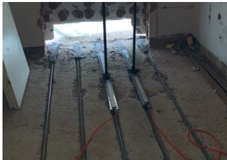
Figure 11. Activation of end-anchored re-bars with infrared heating units (left), RC slab, strengthened with near-surface mounted re-bars (right)
