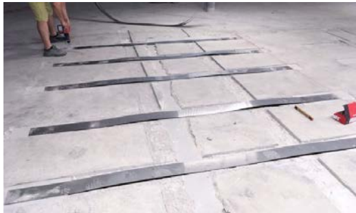
Figure 5. Installation of re-plates in grooves for even concrete surface after strengthening (left), monitoring of heating temperature via re-fer app (right)
