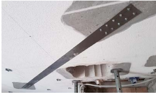
Figure 9. Multi-story building in Goldach (CH): Strengthening of RC slabs over 14 stories due to new openings (left), Residential building in Brunnen (CH): Strengthening of RC slabs due to removal of load-carrying walls, a total of 12 re-plates was installed (right)
