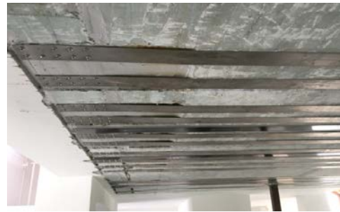
Figure 7. Residential building, Hinwil (CH): Strengthening of cantilever RC slab with 5 m span against deformation due to negative bending moment, 18 re-plates with lengths up to 7 m were used (left), Residential building, Zumikon (CH): Combined use of re-plate and CFRP strips for strengthening of RC slab, installation of 14 re-plates (right)
