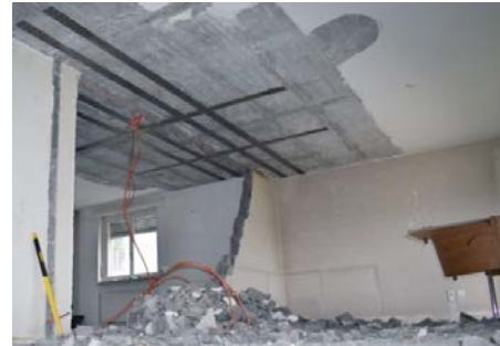
Figure 9. Multi-story building in Goldach (CH): Strengthening of RC slabs over 14 stories due to new openings (left), Residential building in Brunnen (CH): Strengthening of RC slabs due to removal of load-carrying walls, a total of 12 re-plates was installed (right)
