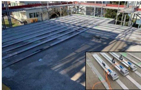
Figure 7. Residential building, Hinwil (CH): Strengthening of cantilever RC slab with 5 m span against deformation due to negative bending moment, 18 re-plates with lengths up to 7 m were used (left), Residential building, Zumikon (CH): Combined use of re-plate and CFRP strips for strengthening of RC slab, installation of 14 re-plates (right)
