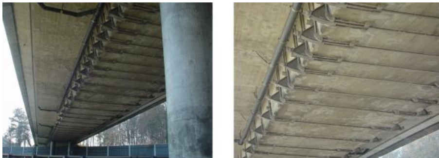
Figure 3: Bridge over the Swiss motorway A1 with shear strengthening.
