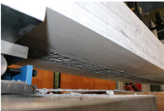
Figure 11. Failure mode of Beam EBR: debonding of the CFRP strip from the concrete surface.
