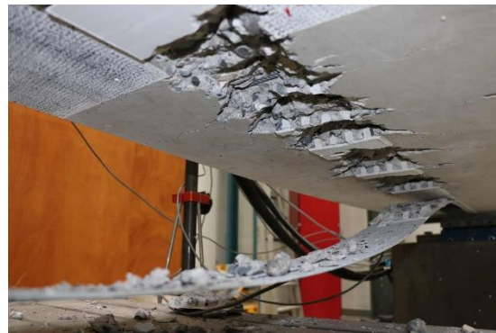
Figure 12. Failure mode of Beam EBROG: debonding of the CFRP strip from the concrete surface with partly concrete cover separation.
