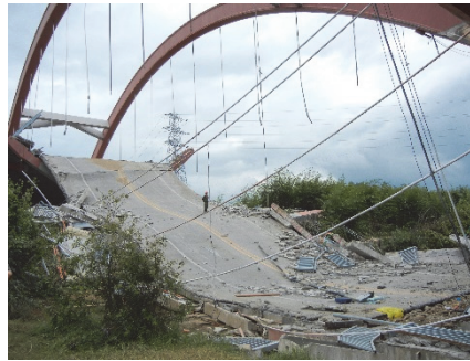
Fig. 7 Gongguan Bridge of Wuyishan, Fujian Province
