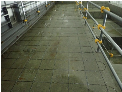
Figure 5. OF cable installation on top
