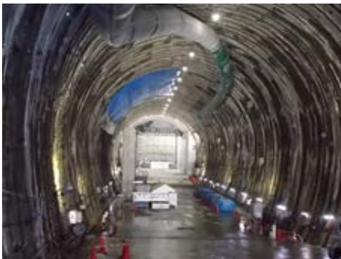
Figure 1. Mock-up of concrete pit in tunnel
