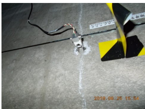
Figure 7. Installed crack gauge
