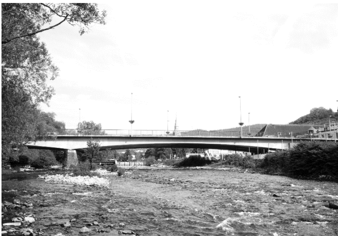
Figure 3. View of the Stennert bridge in Hagen/Hohenlimburg.
