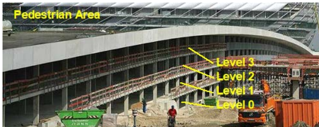
Figure 1. View of the parking garage during construction.
