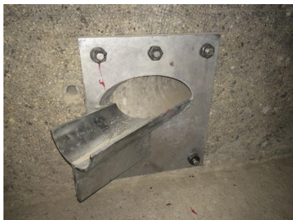
Figure 11. a) Unique steel element made of steel type S235 J2, for the positioning of the anchorage of the post-tensioning cables, b) steel reinforcement detail of the cable anchorage.
