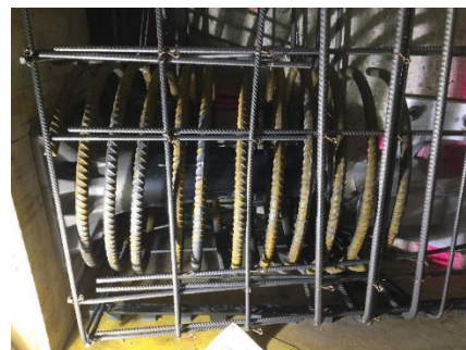
Figure 11. a) Unique steel element made of steel type S235 J2, for the positioning of the anchorage of the post-tensioning cables, b) steel reinforcement detail of the cable anchorage.
