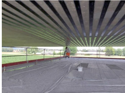
Figure 14. Positioning of carbon fibre reinforced polymer strips (80 mm large, 1.4 mm thick). .
