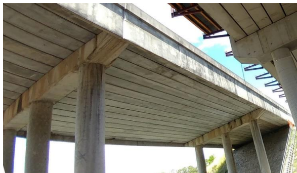
(a) View of the tested bridge span from underneath
