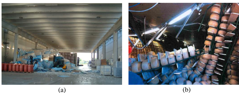
Figure 3. Examples of consequences after the 2012 Emilia earthquake (a) STO and CAP (b) PRO and REA (source: Agenzia regionale per la ricostruzione – Sisma 2012).
