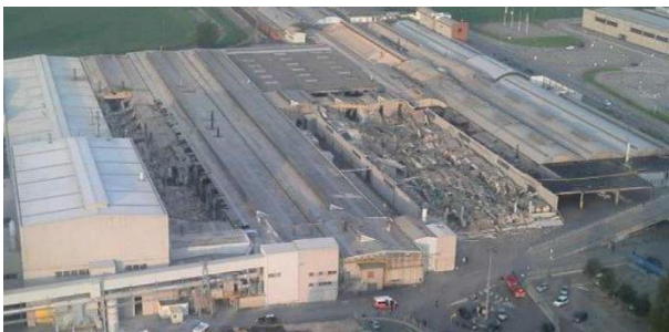
Figure 1. Example of LSB damaged building in Emilia-Romagna (source: Agenzia regionale per la ricostruzione – Sisma 2012).
