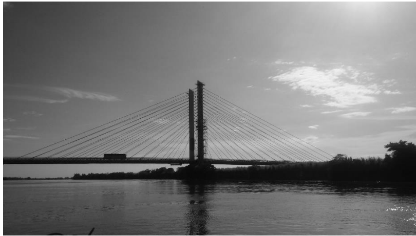
Figure 1. The Papaloapan Bridge.
